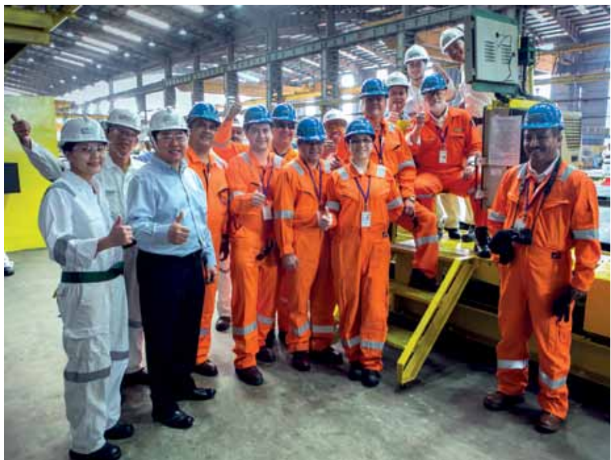
Cutting steel to mark the start of the construction of the first three Grupo R jackup rigs are Mr Chow Yew Yuen (third from left), CEO-Designate and COO of Keppel O&M with Mr Jorge Witte (seated), Project Director of Grupo R, Ms Wong Xin Yi (back row, second from right), Project Manager, Keppel FELS and Mr Roy Tan (back row, first from right), Project Manager, Keppel FELS
